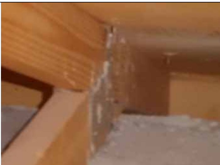
Roof to wall attachment
