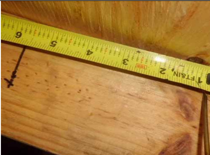
Roof deck attachment
