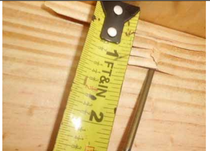
Roof deck attachment
