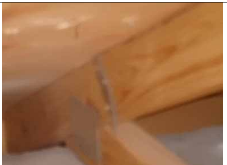
Roof to wall attachment
